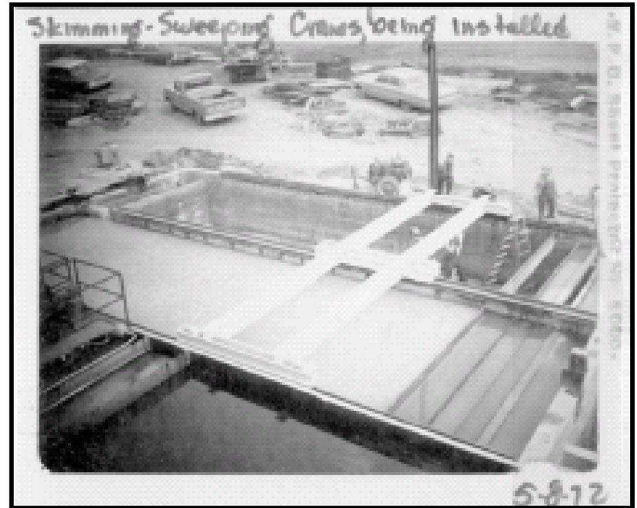
Photo 18 - May 8, 1972 photo. View looking north from WWTP roof.
