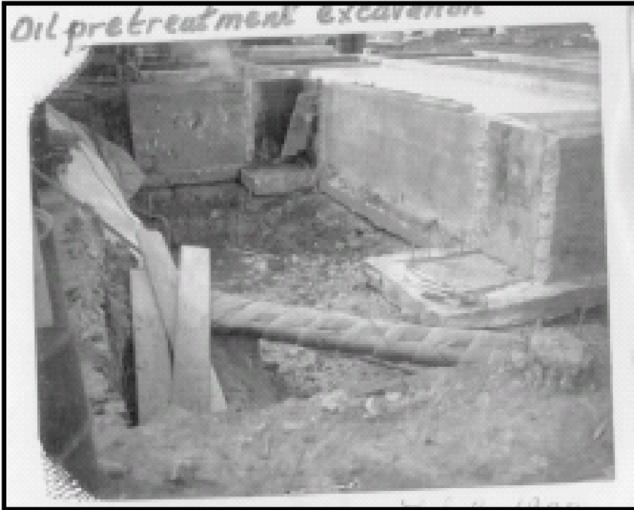
Photo 7 – February 1972 photo. View looking west from east side of WWTP tanks. Note both former (original 4'x4') sump pads and excavation for new EQ tank. Original EQ tank is visible in background.
