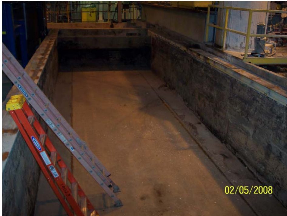
Photo 1 - Building 41, South Settling Basin looking west.
