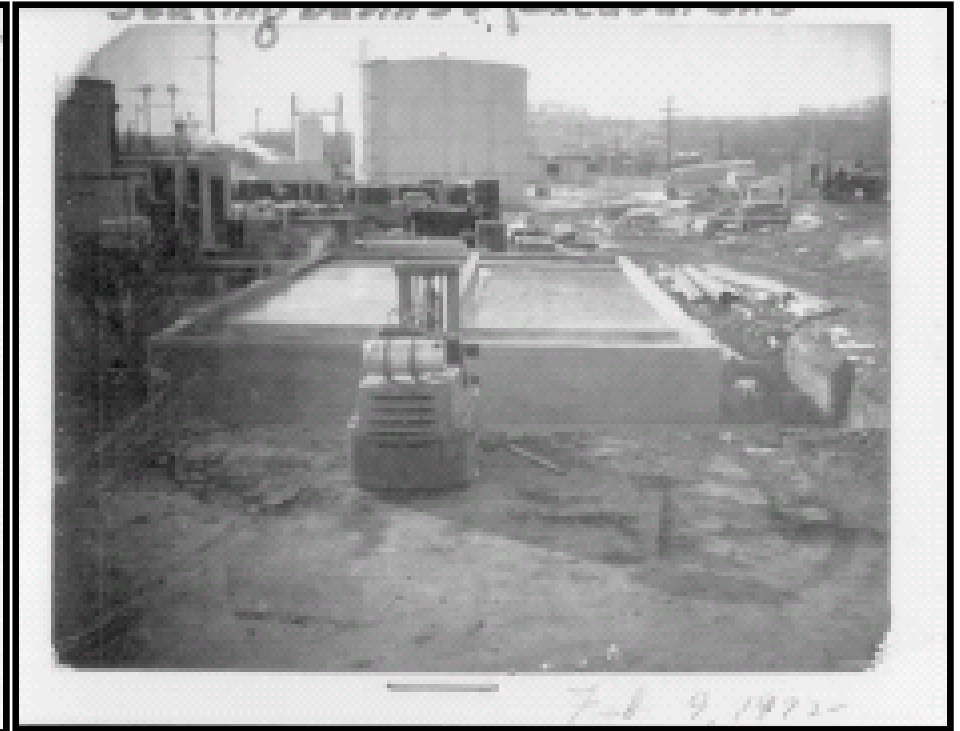
Photo 4 - February 9, 1972 photo. View looking west, east of new settling basins. Note fire protection tank in background and absence of EQ tank.
