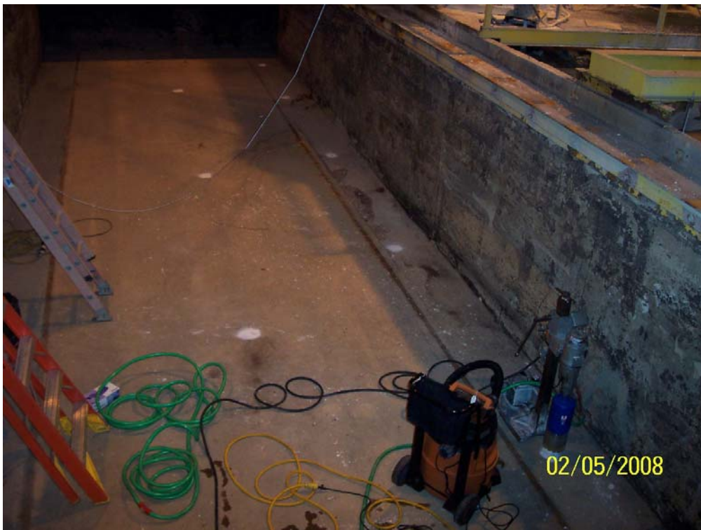
Photo 4 - Building 41, South Basin, looking east. Note soil boring locations in white paint on basin floor.
