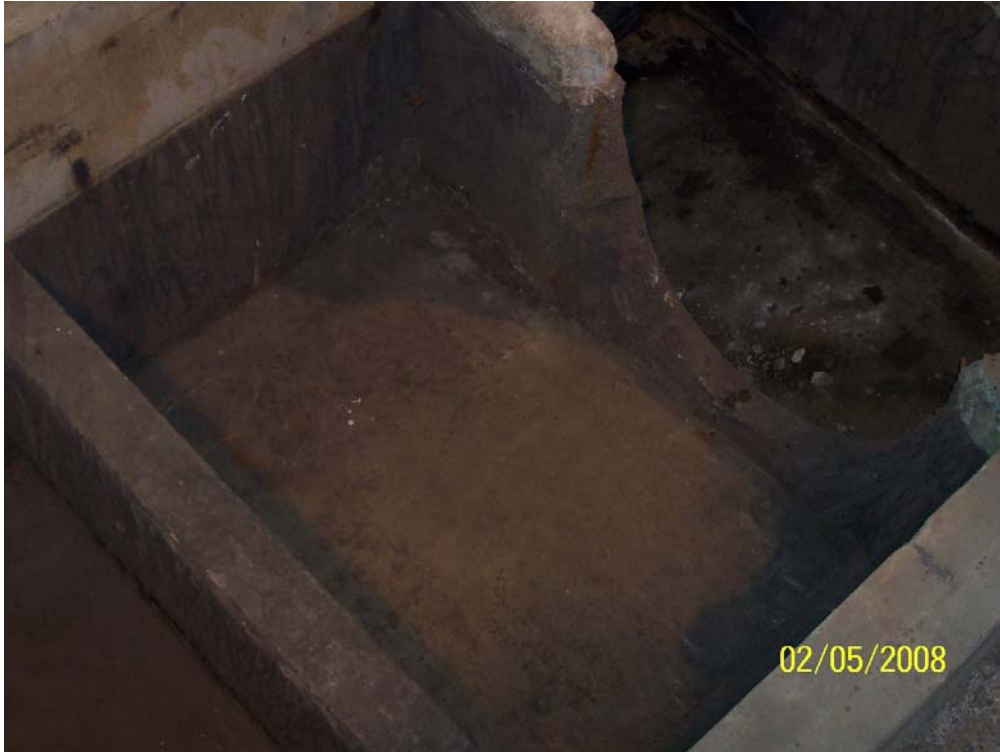
Photo 3 - Building 41, Southern sections of East Basins
